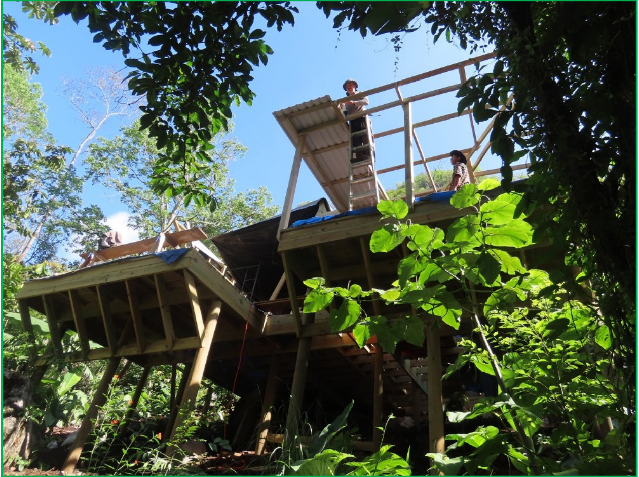
Beginning to install the roofing for the individual decks.
