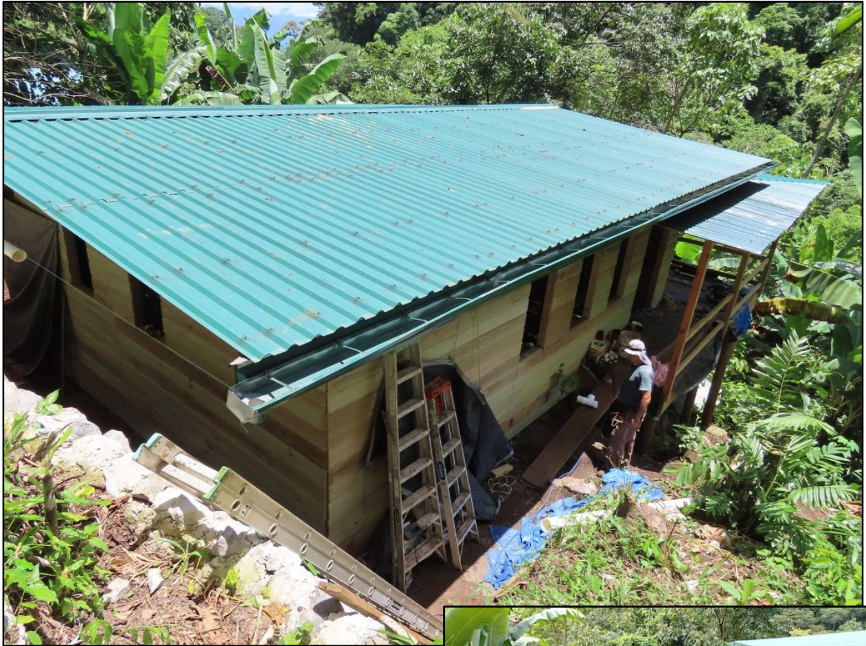
New duplex cabin will be finished by June.
