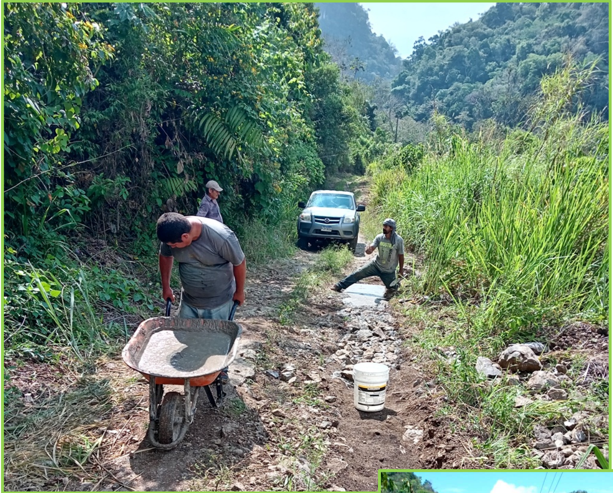
Laying down more cement tracks along the access road.
