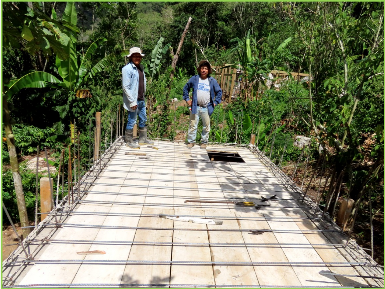
Masons stayed with us for five weeks, carrying out various projects. This rainwater collection tank will hold over 15,000 gallons and will be fed by the first duplex cabin.
